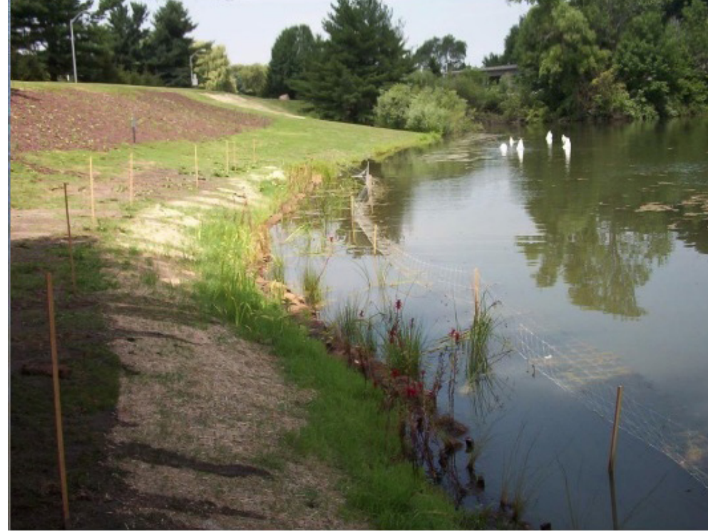
Coir log installation and 2-3 weeks after installation of plantings
