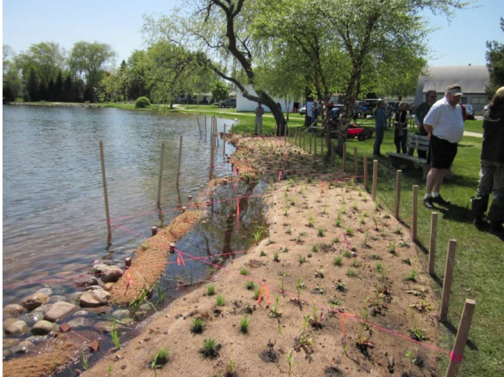
Initial installation in small pond (no slope present). Native plugs installed in erosion blanket.
