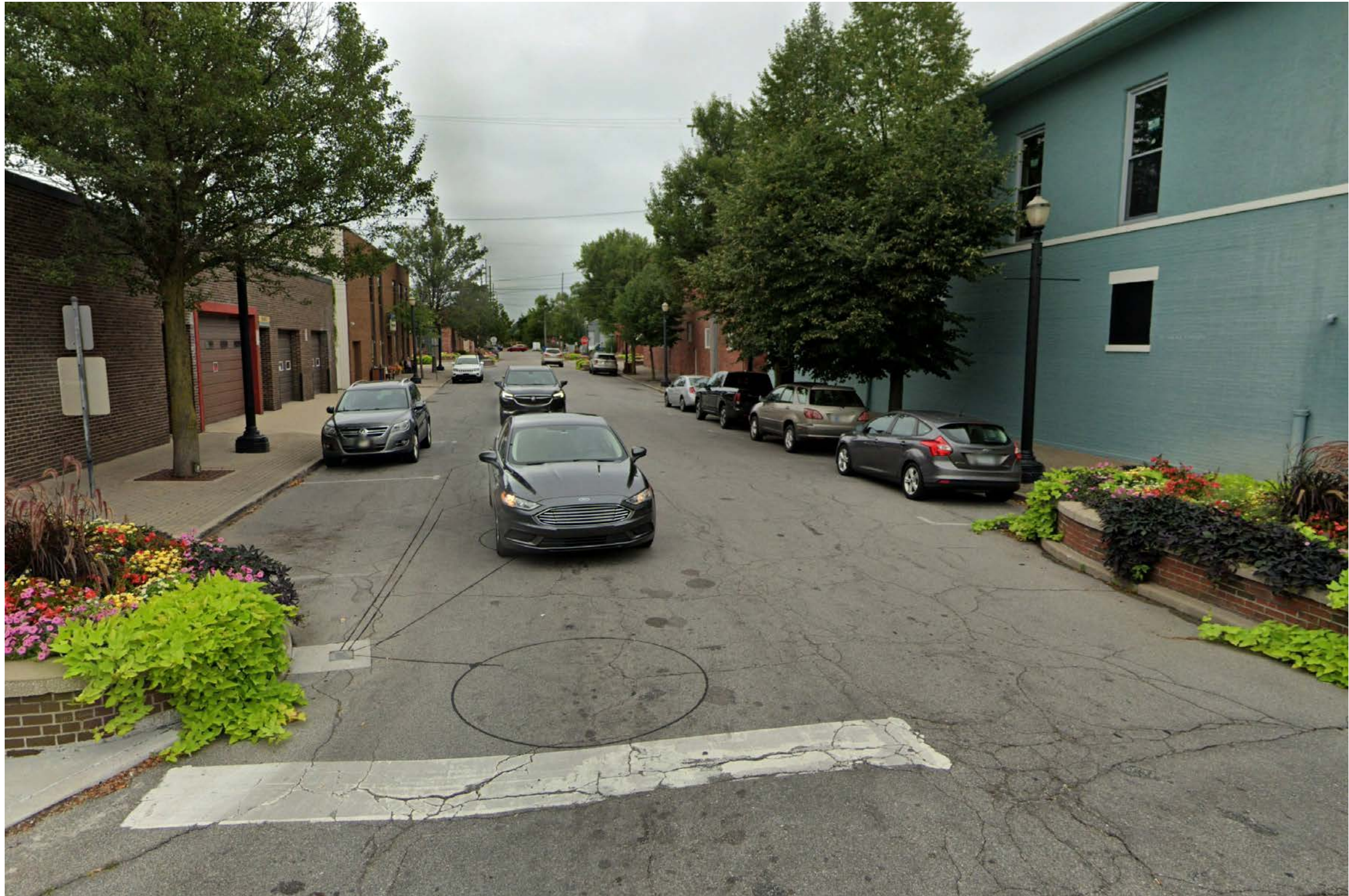
Existing Conditions - Midblock C
